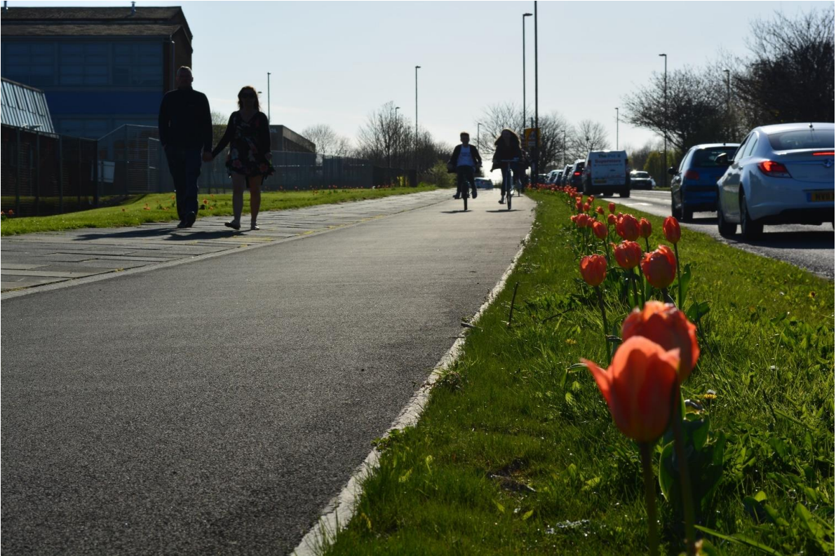
Figure 10 Path near a secondary school, single surface with indicative change in materials (Sustrans)
