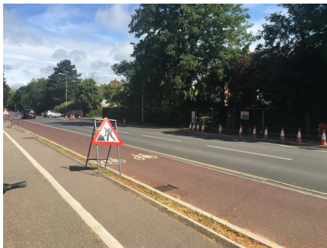
Figure 20 Unidirectional Cycle Tracks under construction, Cambridge 2016
